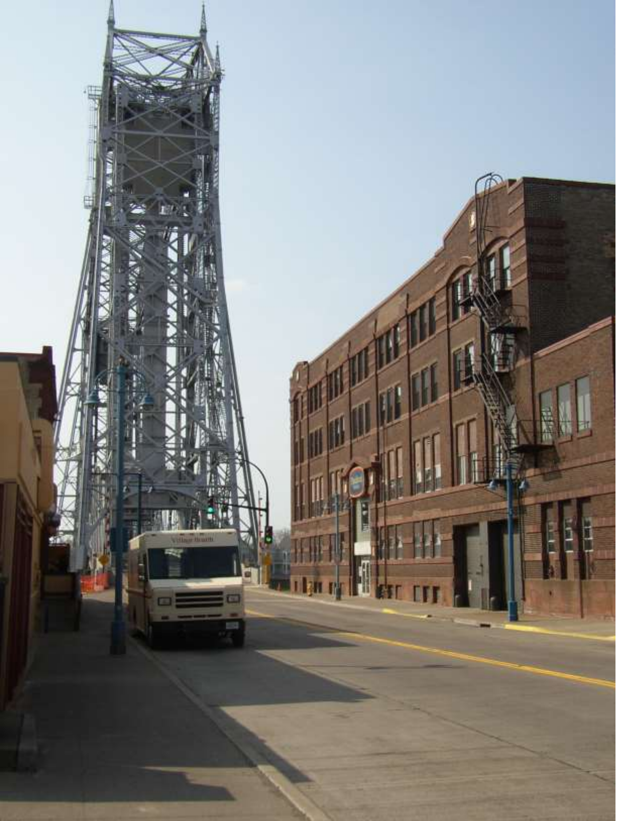
Aerial P Building
